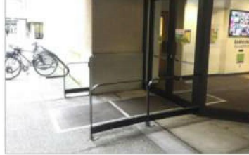
Figure 16: Outward-opening power-operated doors with cane-detectable guards
